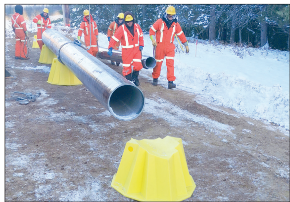
Figure 5b: An RS Pole on Pole Stands
