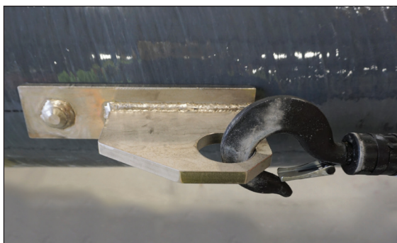
Figures 11a and 11b: Jacking Plates Aligned in the Direction of the Assembly Force and Tight Against Pole Wall
