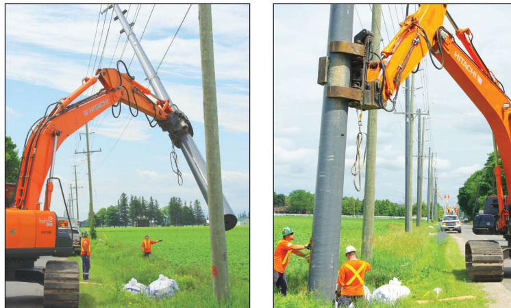
Figures 25a and 25b: A Pole Setter Setting a Double Circuit 44kV Pole During an Outage
