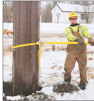
Figure 27: RS Poles Can Be Turned Easily Using a Pole Cant
