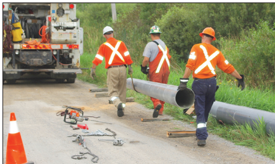
Figures 4a and 4b: Small Modules Being Unnested and Laid Out for Assembly
