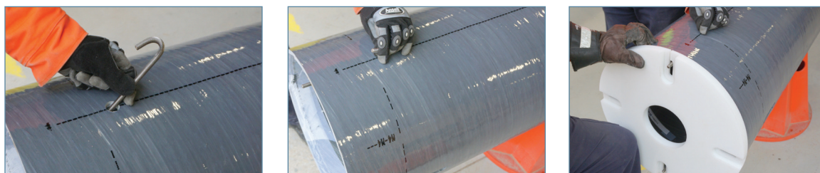
Figure 19a, 19b and 19c: Installing a J-Bolt into the Pre-Drilled Hole and Positioning the Base Plate
