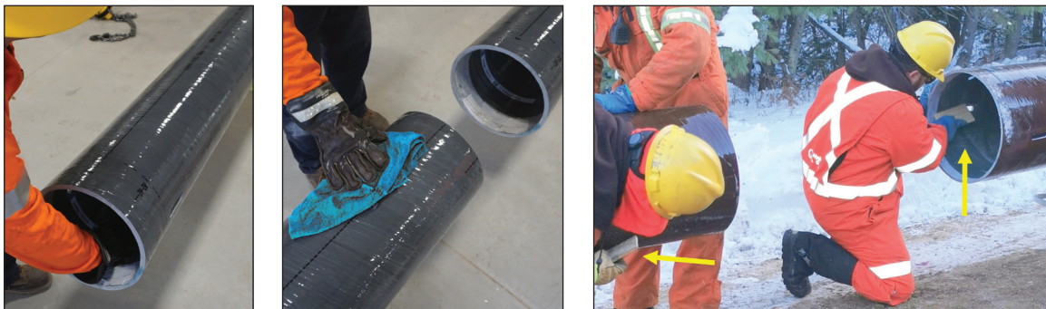
Figures 7a, 7b and 7c: Wiping the Inside Surface of the Upper Module and the Outside Surface of the Lower Module
