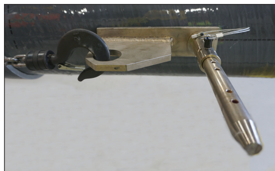
Figures 11a and 11b: Jacking Plates Aligned in the Direction of the Assembly Force and Tight Against Pole Wall
