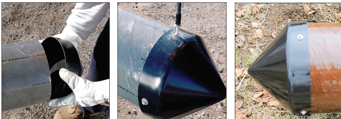
Figures 21a, 21b and 21c: Positioning and Installing the Top Cap
