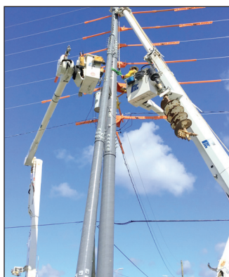
Figures 30a and 30b: Base Module Being Replaced Using Live Line Techniques
