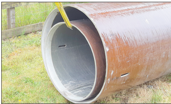
Figures 3a and 3b: A Derrick Boom Truck Lifting Up and Outwards to Unnest Modules and Prevent Scratches
