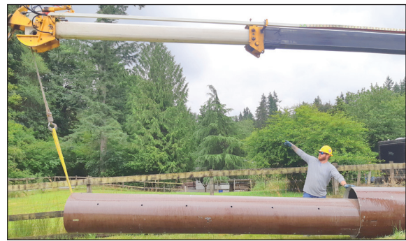
Figures 3a and 3b: A Derrick Boom Truck Lifting Up and Outwards to Unnest Modules and Prevent Scratches
