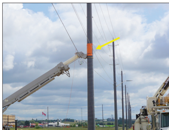
Figure 23: Temporary Rubber Matting to Protect the Pole Surface From the Boom
