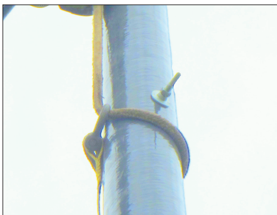
Figure 22: Temporary Through Bolt to Prevent Sling Slippage
