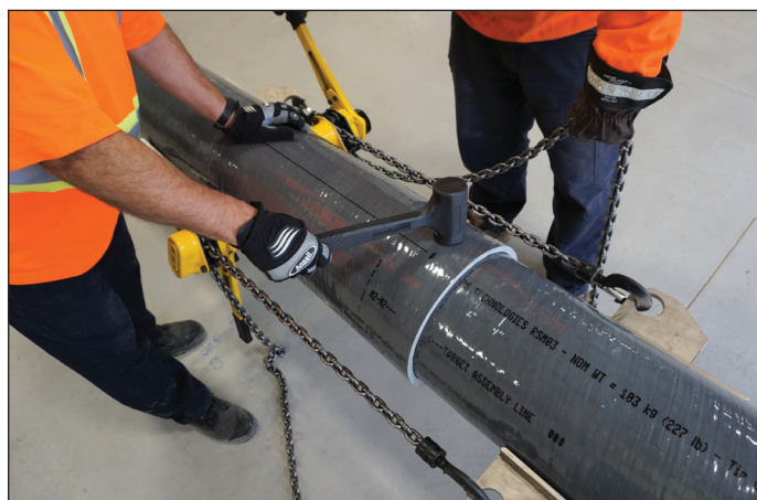
Figure 13: Alleviating Static Friction Using a Dead Blow Mallet
