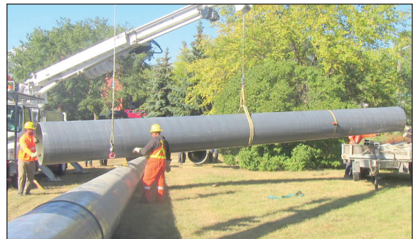
Figures 4a and 4b: Small Modules Being Unnested and Laid Out for Assembly
