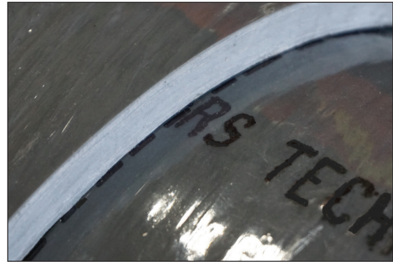
Figure 15: Example of a Slip Joint Assembled to the Circumferential, Pre-Marked Target Assembly Line
