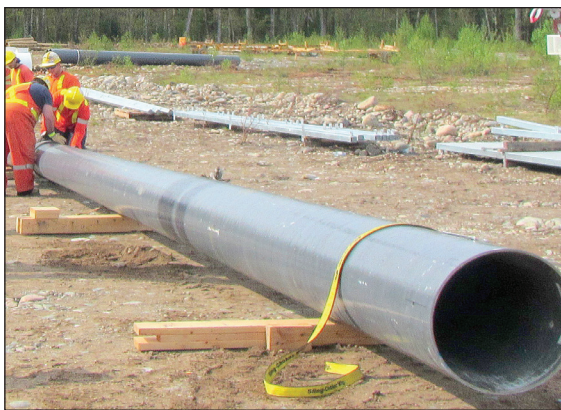
Figure 5a: An RS Pole on Wood Dunnage
