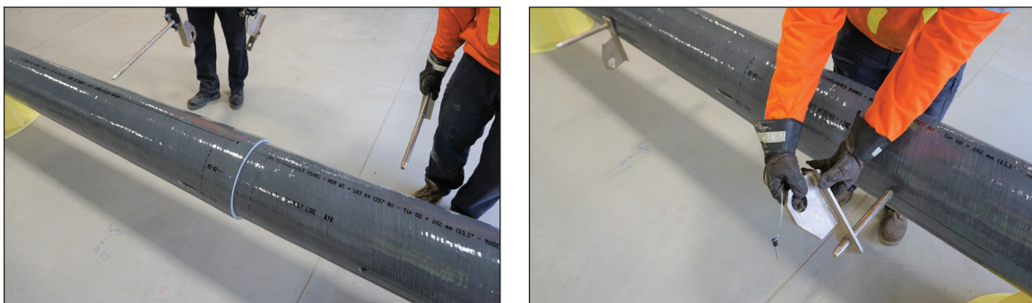
Figures 9a and 9b: Inserting the Jacking Bars and Adding the Jacking Plate
