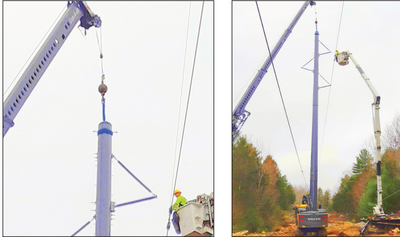
Figures 24a and 24b: Crane With a Choker Sling Installing a 95 ft. [29m] Pole for a 115kV Circuit
