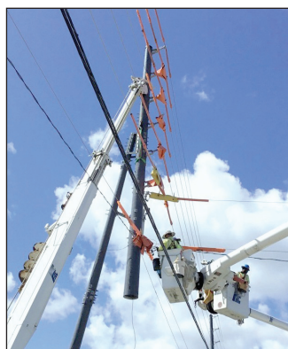
Figures 30a and 30b: Base Module Being Replaced Using Live Line Techniques
