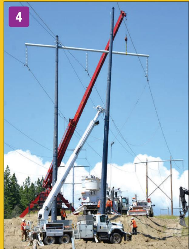
Process to replace wood framing with composite poles.
