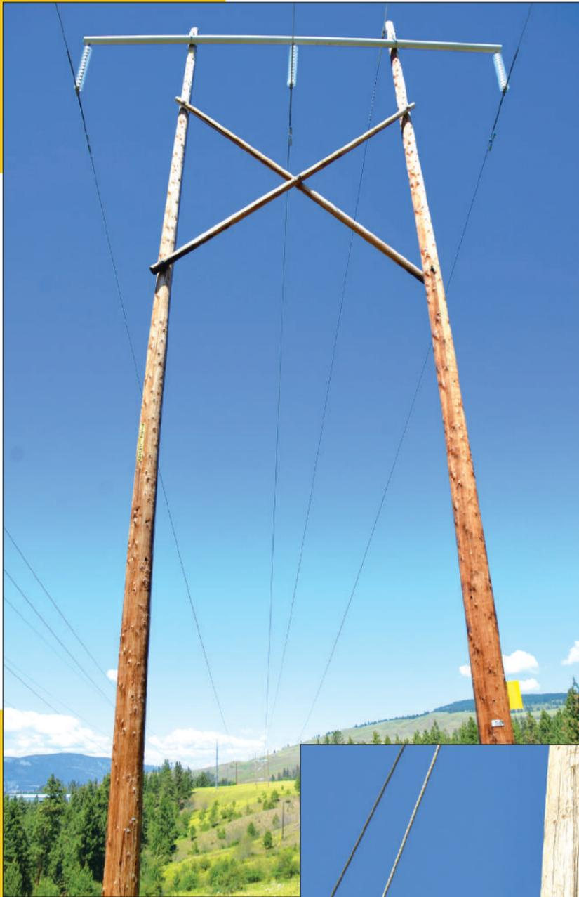
FortisBC, a utility operating in the west coast province of British Columbia, conducts maintenance assessments of its overhead lines on an 8-year cycle. This includes both below grade and above grade inspections of each structure. Apart from checking sample wood poles for issues such as moisture penetration, visual assessment is also performed on structures, cross-arms, line hardware and conductors.
