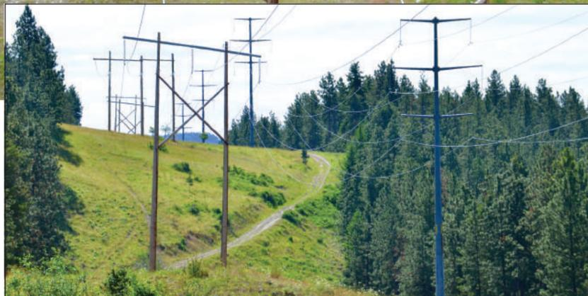
230 kV line (left) running from Lee Substation in Kelowna to Vernon has suffered woodpecker damage to some poles and was selected to test new composite pole.
