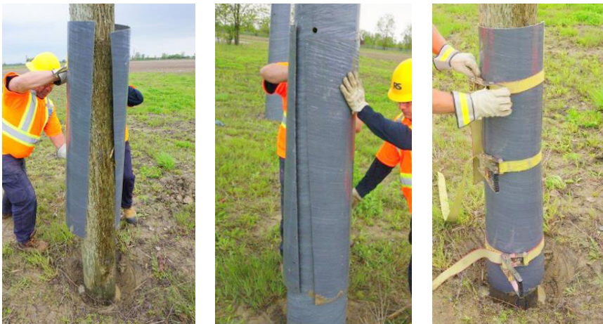
Figure 11: Temporarily holding the primary shield in place on the destination pole with ratchet straps.
